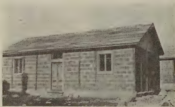
Temporary barracks for returned refugees built of brick, to resist the cold in this mountain climate, more than 3,000 feet above the sea
